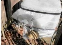
13) The A/C system was not turned on due to cold weather. Did note the compressor was covered in plastic, which can trap moisture and damage the unit. Recommend removing the cover. The system should be thoroughly evaluated by a qualified technician prior to closing. (Please also see Attic 2 section)
