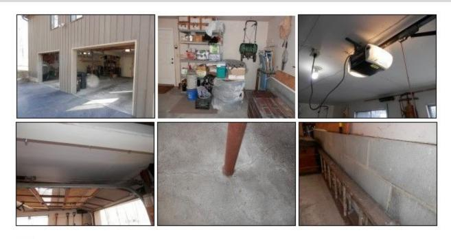
11) . Garage doors, safety cables and the auto-reverse function performed as expected. The garage ceiling, walls and windows were also in serviceable condition. The concrete floor showed minor pitting from salt and other ice melting chemicals over the years. A garage door torsion spring is sagging and worn; this is a safety hazard. Recommend a qualified technician evaluate and repair or replace.
