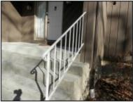
4) The front entry stoop and landing were in acceptable condition. However, a railing was loose, which is a hazard. It should be repaired or replaced by a qualified contractor.
