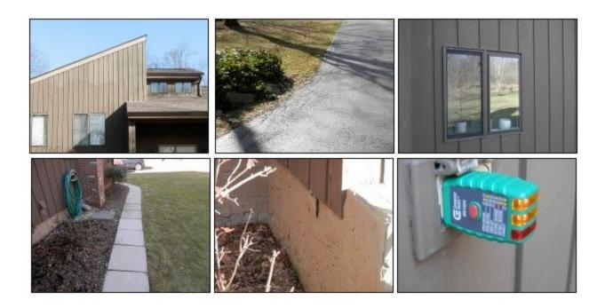
1) The exterior grounds, foundation walls, grading, walkways and windows were in acceptable condition. Outside GFCI outlets tested and operated as designed.. Did note some paint peeling in small areas of the exterior wood siding and trim. This could result in the wood rotting if left unattended. The driveway was graded away from the home and was in acceptable condition. Noted minor asphalt cracks in some areas which could become a problem over time. Recommend monitoring and routine maintenance.
