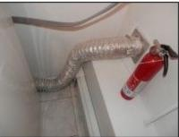
32) A note on dryer venting: an accordion-type flexible vent hose can trap lint and is susceptible to kinks or crushing. A corrugated semi-rigid metal duct is preferred. Exhaust hoses and vents should be routinely cleaned.
