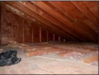
8) Stored materials prevented a complete inspection of the attic. I recommend a follow-up inspection once attic obstructions are removed. Unable to determine if roof soffits were obstructed. Inadequate attic ventilation may result in high attic and roof surface temperatures, reduce the life of the roof covering and insulation materials and increase cooling costs. A qualified contractor should evaluate and repair or replace as necessary.
