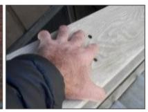
2) The upper deck footings, railings, and handrails showed signs of wear. The steps had open risers. This could be a safety hazard for children. Unable to observe the concealed area below the lower deck to examine the footings, ledger boards or joists. The proximity of deck benches to the edges of the lower deck may present a safety issue. Consider installing railings to prevent accidental falls. Recommend a qualified contractor evaluate and repair or replace deck components as necessary.
