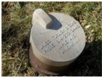
17) The drilled well sanitary cap is too low to the ground and improperly sealed. This is a health and safety issue because the cap is supposed to prevent contaminants from getting into the water supply. Recommend having a qualified contractor evaluate the well system components prior to closing. Also suggest asking the owner for any well maintenance records.
