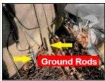
20) Noted the underground service entrance conductor was rated for 150 amps and appeared to be securely fastened to the side of the home. Also noted 2 ground rods securely fastened.
