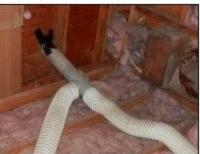
7) The whole house attic fan operated satisfactorily. Did note two attic exhaust fan hoses joined at a "T" connection leading to a single exterior vent. This could allow one of the bathroom's exhaust to return to the other bathroom instead of exiting thru the attic vent. Also, the hose is attached to the sidewall vent with duct tape and is not sufficiently secured. Recommend a qualified contractor evaluate and repair or replace as needed.
