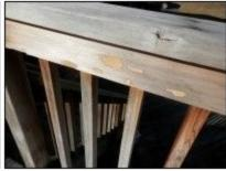
3) Shrubs were in contact with wood siding. While there is no evidence of moisture intrusion, over time foliage can stain and/or degrade the siding. Recommend pruning or moving the shrubs. The wood siding and deck showed evidence of repairs from minor insect damage. Recommend evaluation by a qualified pest control company.
