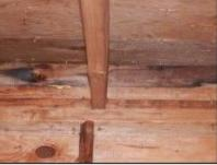
9) Stained sheathing and rafters with low moisture readings are an indication of past water intrusion. Despite recent heavy rains and snowfall, these areas were dry on the day of the inspection. These leaks may pre-date the existing roof surface. Recommend cleaning and monitoring these areas in the future to determine if active leaks exist.
