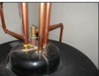
19) The hot water heater is part of the boiler system and operated as designed on the day of the inspection. It has a properly installed temperature relief valve and extension. For more in how indirect water systems work: <a href="CLICK HERE">CLICK HERE</a>.
