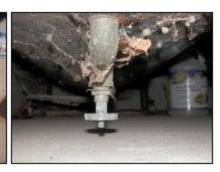
15) Stored items obstructed the view of the oil storage tank. However, did observe that the fuel oil components worked properly, and no leaks were detected on the day of inspection. Expected effective life of an oil storage tank is 20-25 years. This tank appears to be midlife or older.
