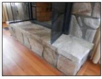
26) A Level 1 inspection was performed. The fire box condition was acceptable and the damper performed as designed. Did note an area of concern: there were gaps between fireplace metal frame and the stone surround. Given the proximity of the wood floor and adjacent curtains, this could create a fire hazard. Recommend a Level II inspection of all fireplace components by a qualified chimney sweep technician prior to closing.
