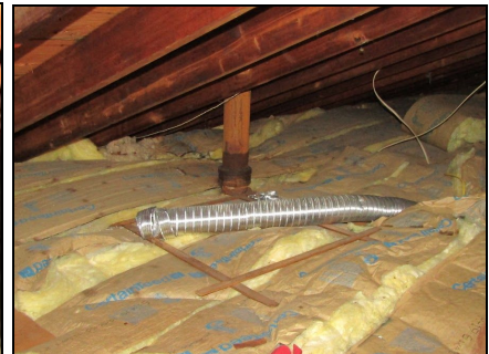
Bathroom Exhaust Vent Pipe
